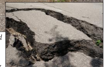
The road here has shifted vertically 4 feet
