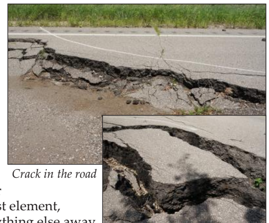
The road here has shifted vertically 4 feet
