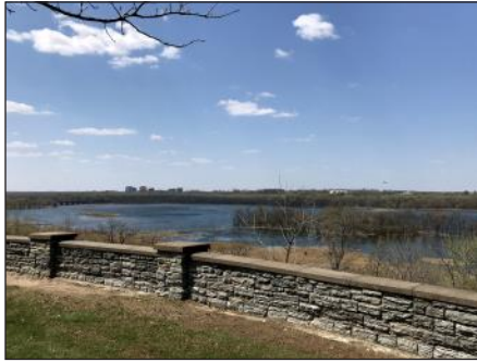
A portion of the WPA stone wall at the Big River Regional Trailhead in Mendota, MN. The MSP airport is located across the river.
