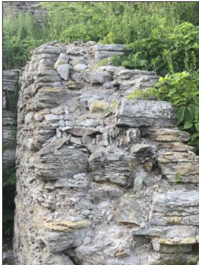
Three-foot thick (basement?) wall constructed with both outer and inner stone blocks and a core of smaller rubble stone. Cathedral Hill area of Saint Paul
