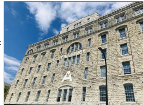
The Pillsbury A Mill (1881) was constructed from stone quarried onsite and along the river banks.
