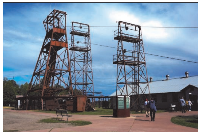
Soudan Mine Headframe
