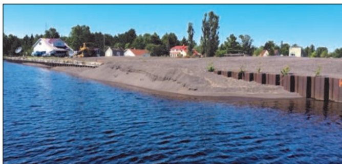
Stamp sands overflowing the breakwater at Big Traverse.
